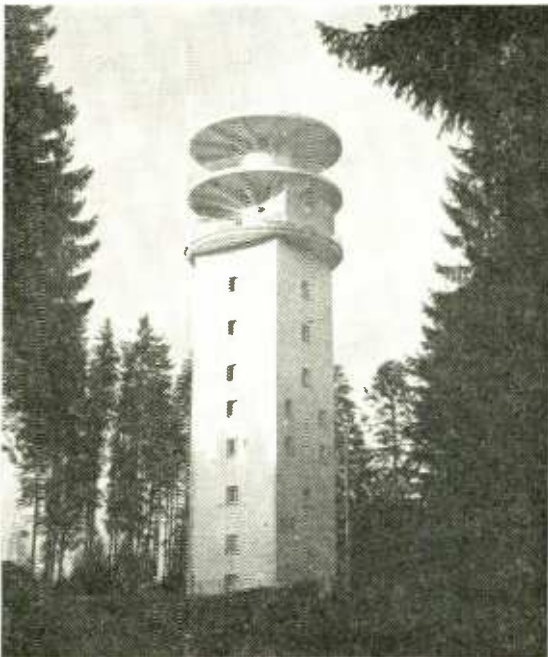
Television relay station in the Paris-Strasbourg chain at Dabo la Hoube in the Jura, constructed by Cie Generale de Telegraphie Sans Fil.
