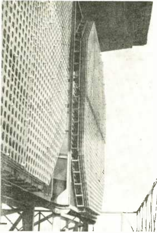
Pair of 30-cm relay aerials with electromagnetic lenses, built by Cie Generale de Telegraphie Sans Fil.
